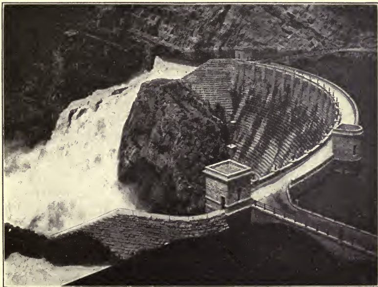
ROOSEVELT DAM, ARIZONA
